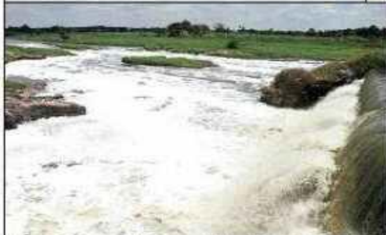
Musi flows with industrial effluents and rain water at Pirzadhiguda, Uppal
